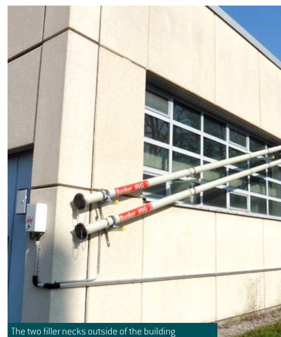
The wood gas is produced in the gas reactor.
