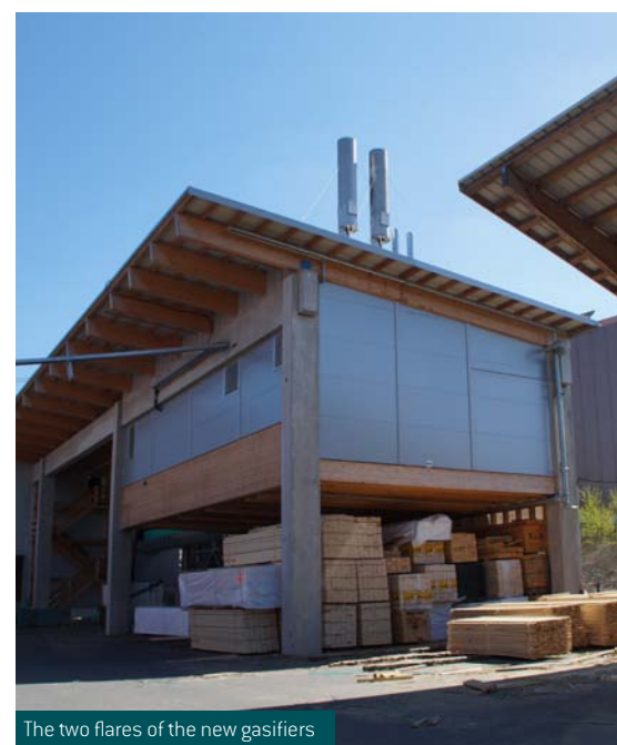
Focus on wood – Also in energy production.
