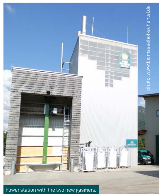
After modification: now two Burkhardt Gasifiers supply one CHP
