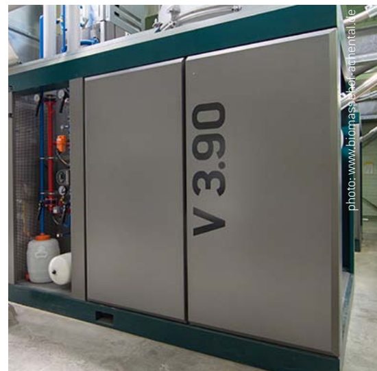
After modification: now two Burkhardt Gasifiers supply one CHP
